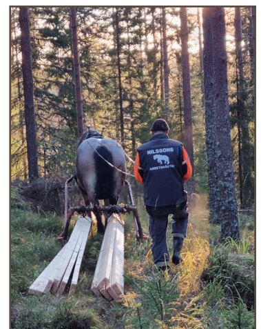
Working horse on Finnvägen again, but this time for laying out duck boards.
